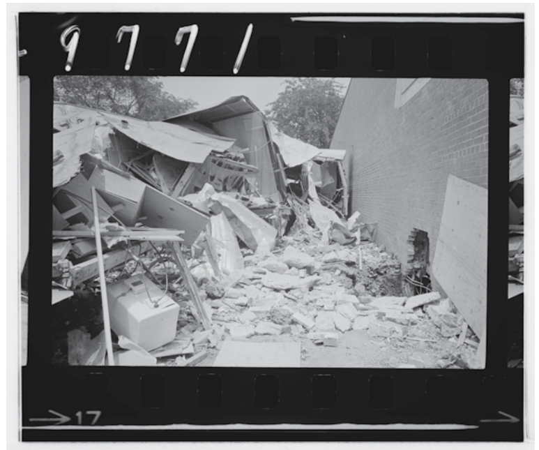
Bomb damage to Gaston Motel in Birmingham, AL, 1963. Birmingham was unofficially named "Bombingham" for the number of bombings taking place there.
