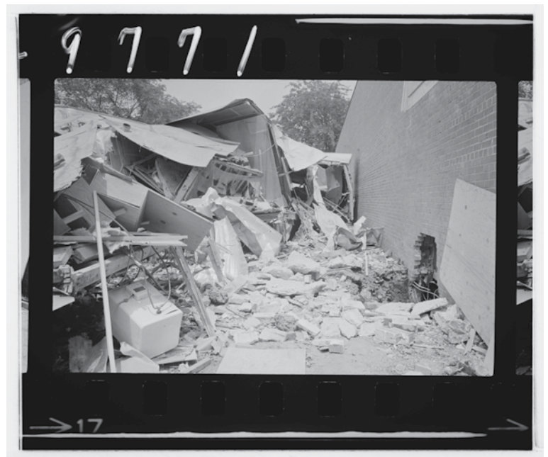
Bomb damage to Gaston Motel in Birmingham, AL, 1963. Birmingham was unofficially named "Bombingham" for the number of bombings taking place there.
